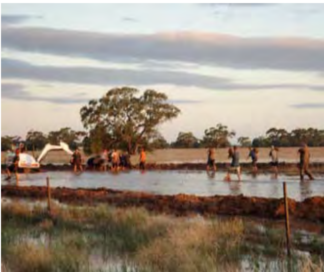
△ Building a levee bank at Wycheproof
