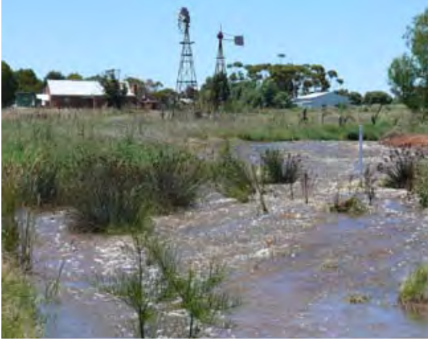
△ Flood water spilling out of the Donald Main Channel at Corack township. The Wimmera Mallee pipeline had just superseded the old open channel system. VicRoads had removed the bridge at Corack on the Donald-Swan Hill Road creating a block in the channel. Flood water caught by the channel through all districts right down from south of Donald, was heading north and filling here.
