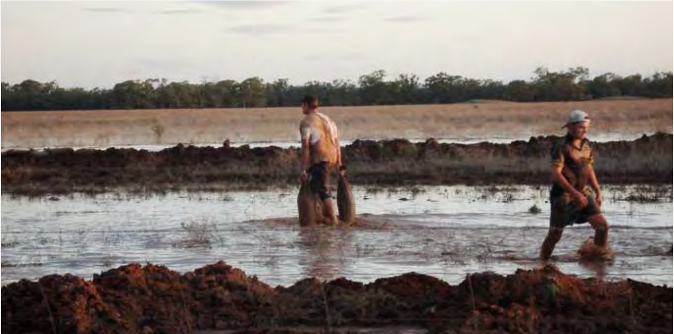
△ Levee bank construction, Wycheproof.
