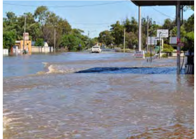
△ Locals try to cross the bridge over the Richardson River.
