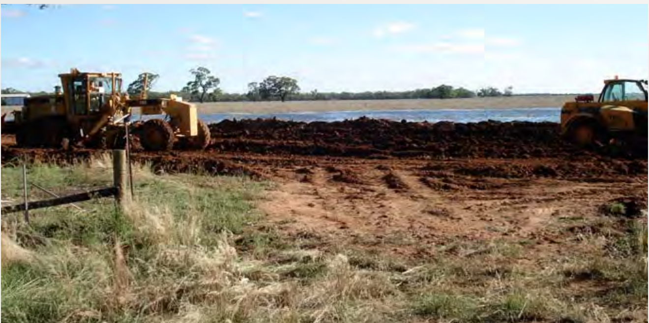
△ Levee bank construction, Wycheproof.
