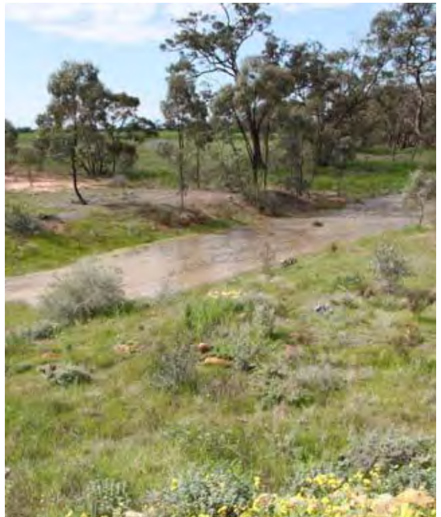
△ Tyrrell Creek about to go under the bridge at Warne on the Calder Highway.
