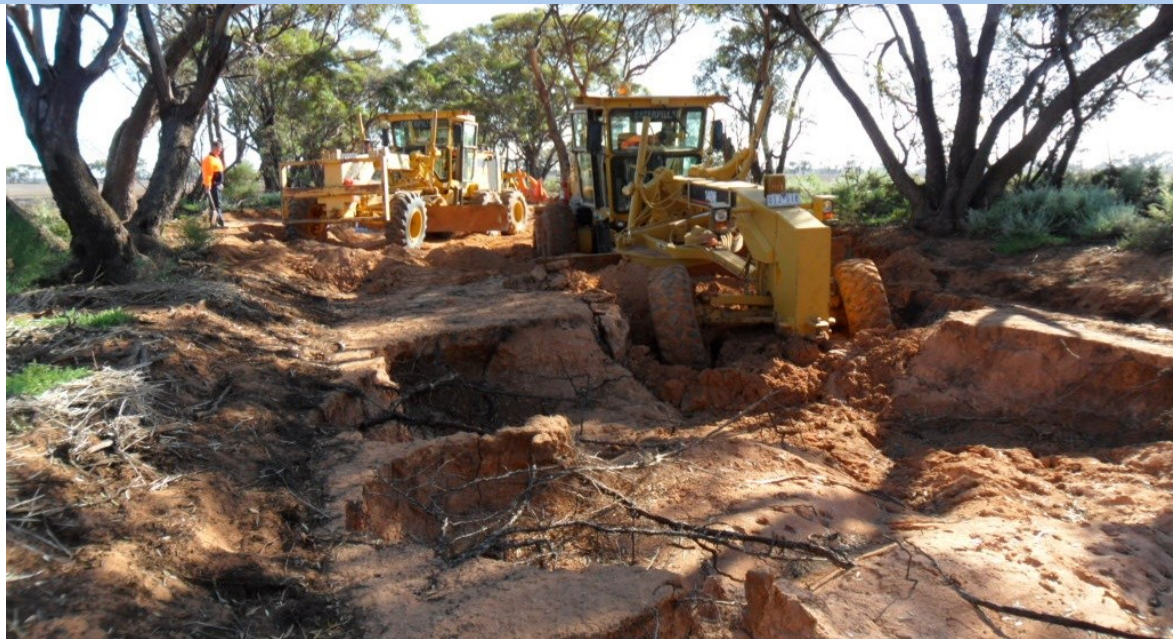
Crews begin work on a flood damaged road
