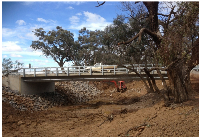
The bridge has been rebuilt using disaster grant funding
