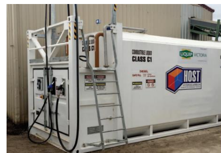
A HOST Self Bunded Tank fitted with a custom pumping & dispensing solution by Liquip Victoria sourced from Appendix D3
