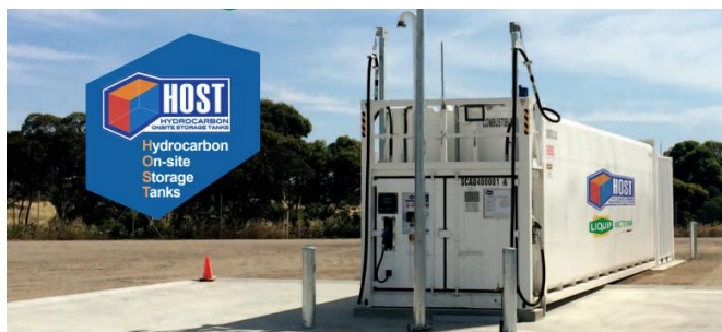
A HOST Self Bunded Tank fitted with a custom pumping & dispensing solution by Liquip Victoria sourced from Appendix D3
