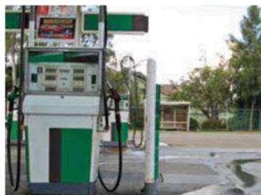
Picture shows a defective forecourt design with oils and fuels discharging directly to the street drain.
