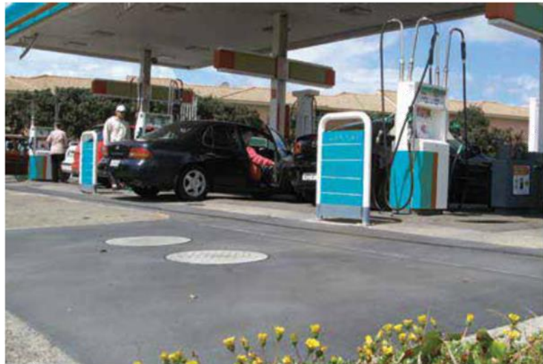
Petrol forecourt and surrounds at a busy metropolitan petrol station rendered compliant. The catchment consists of a grated drain encompassing the complete perimeter of the under-sized canopy. Surface water and forecourt runoff drains to the Puraceptor located under the two trafficable covers in the foreground.
