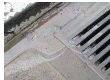
Unseemly & highly visible hydrocarbons polluting the stormwater. The concentration in the picture is in excess of 10ppm
