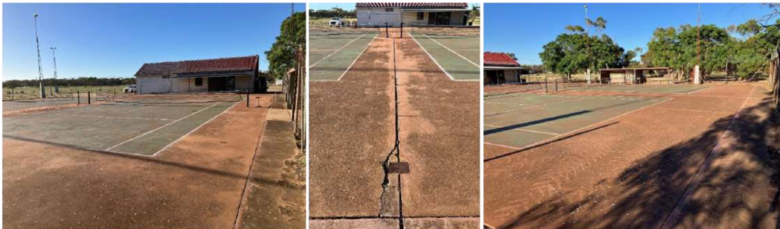
Nandaly. Repair and resurface both courts shown
